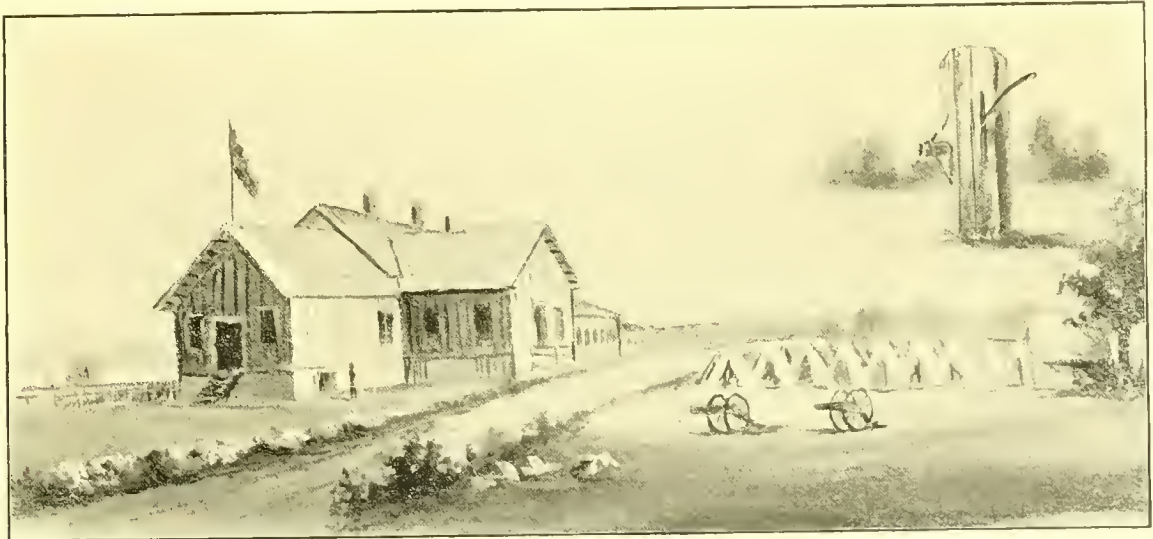
Old Camp Curtin Hospital.
